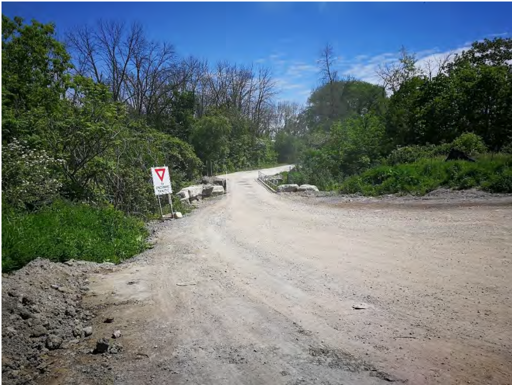
Photo B13: Road Bridge area (looking east)
