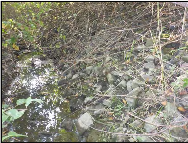
Photo 11. Location 10. Reach S2. Rip-rap protection along lower bank. September 28, 2018.
