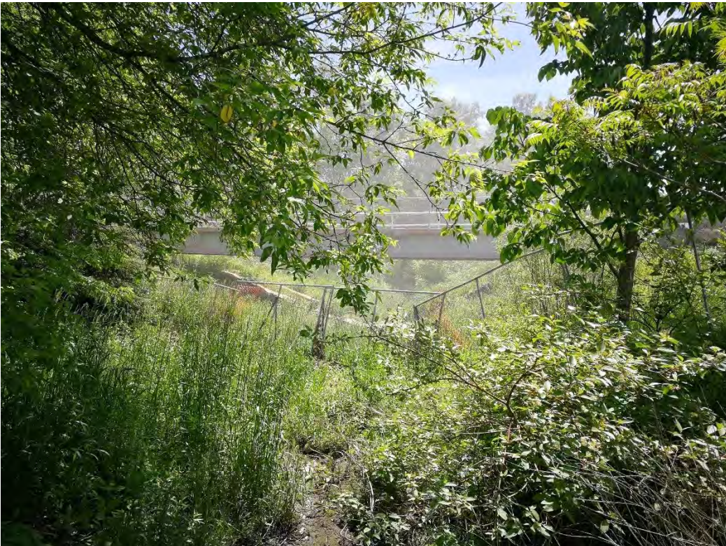
Photo B12: Creek conditions at north of Bridge (looking south - downstream)
