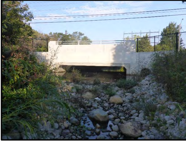
Photo 1. Location 1. Reach S3. Upstream view of designed cobble lined channel and Lakeshore Road E culvert. September 21, 2018.
