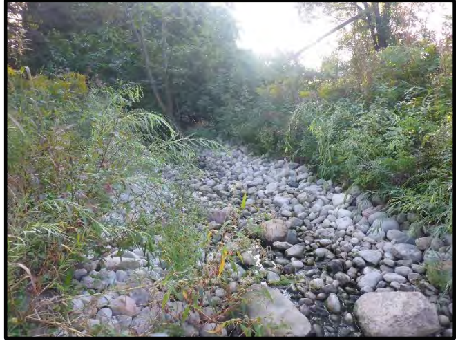
Photo 2. Location 1. Reach S3. Downstream view of designed cobble lined channel. September 21, 2018.
