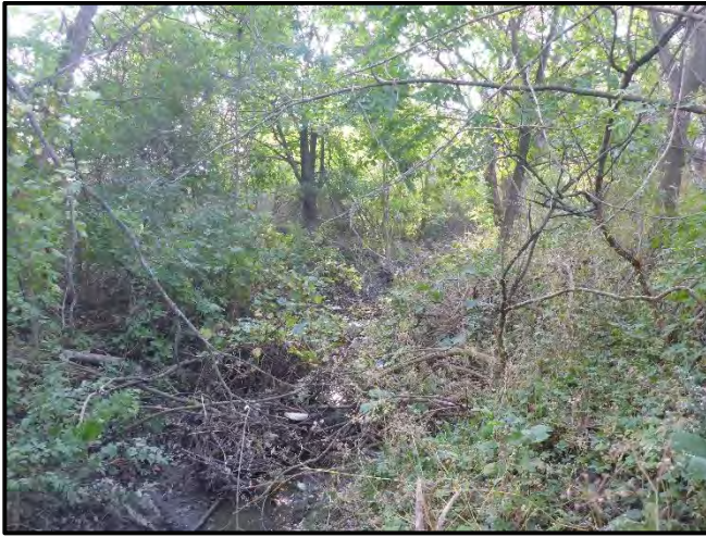
Photo 9. Location 8. Reach S2. Downstream view of woody debris jam. September 28, 2018.
