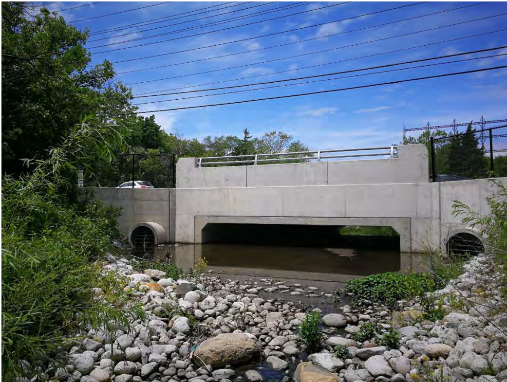
Photo B1: Creek and Concrete Culvert at Lakeshore Blvd (looking north - upstream)
