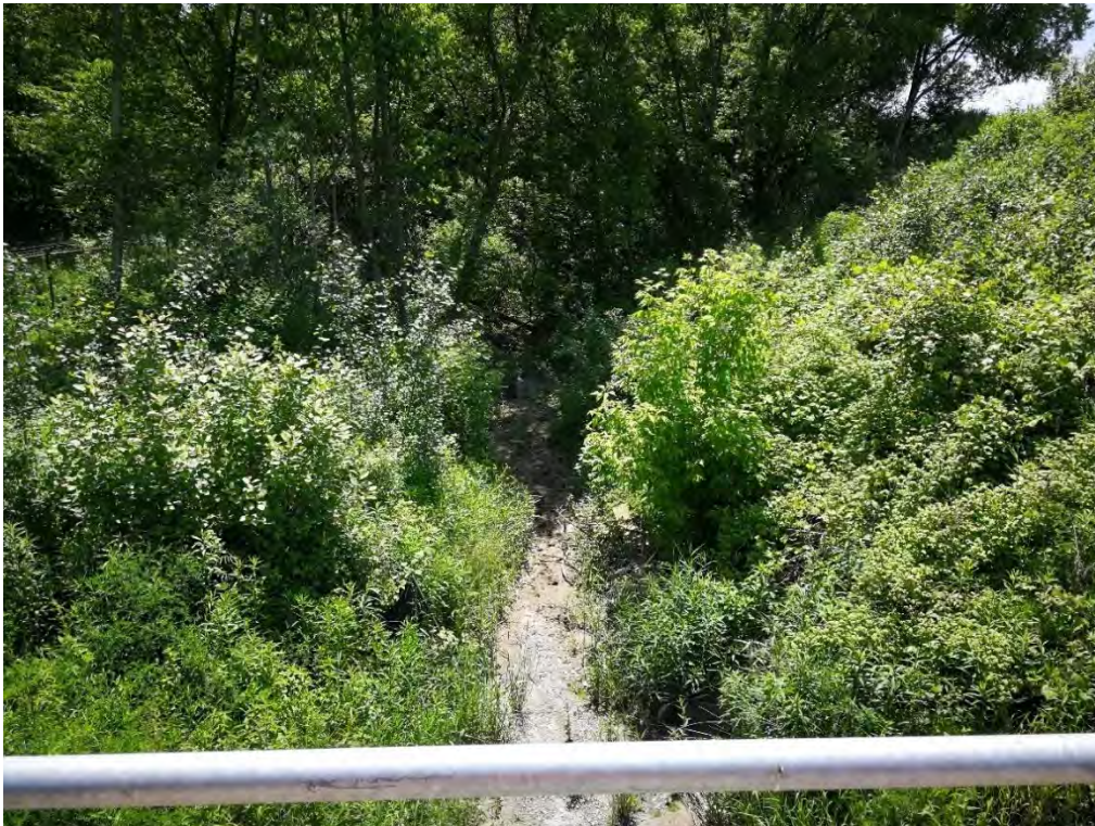
Photo B16: Creek and slope conditions to south of bridge (looking south from bridge – looking downstream)
