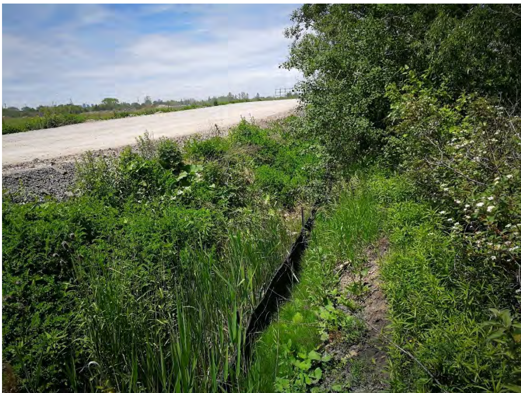
Photo B18: Ditch between Creek and Road at south part of Reach S2 area (looking north - upstream)
