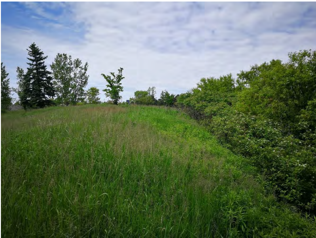
Photo B10: Top of slope conditions to west of Section N-N (looking west)
