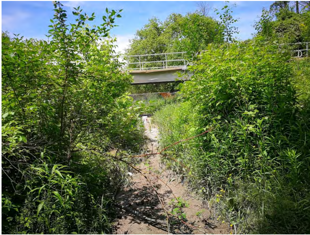
Photo B15: Creek conditions to south of bridge (looking north - upstream)
